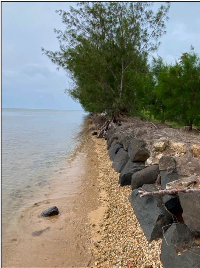
Fig. 9. Riprap systems, Tubuai. Personal photo (12/2020).
